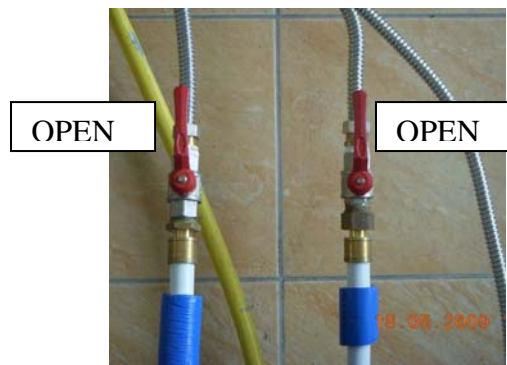
Figure 2 – Taps of the cooling system of the chamber.
